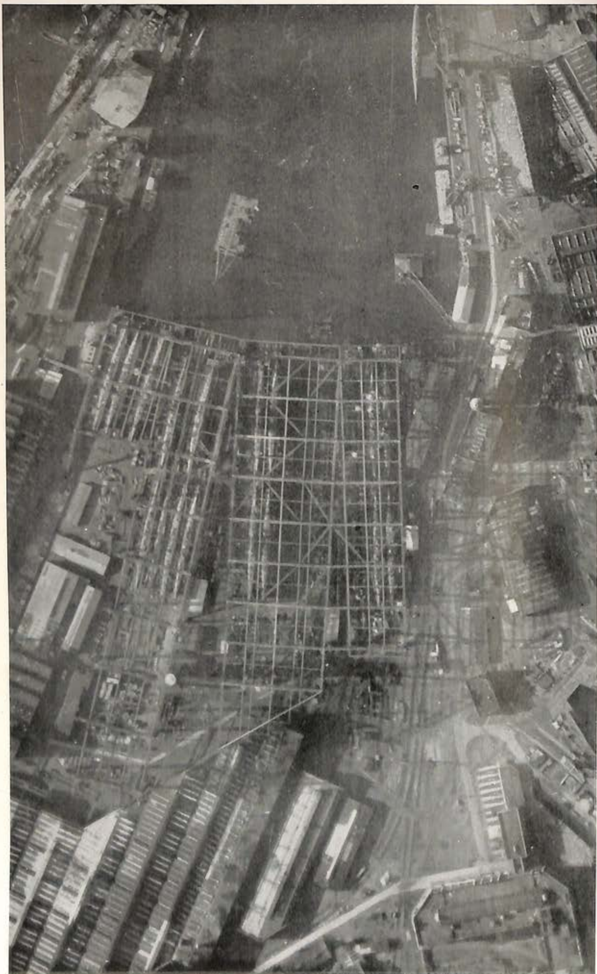
The above photograph, taken during December, 1944, shows the new type XXI U-Boats. These were assembled very quickly from prefabricated sections. Although the sections were made at a number of points, there were only three assembly yards. The Blohm and Voss Yard, seen above, was one.
