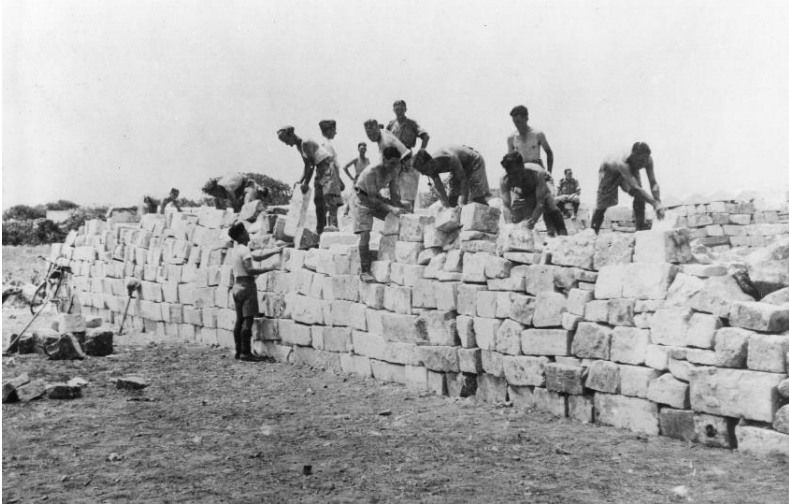
Protective aircraft pens under construction at Takali; they were built entirely by hand using a variety of materials, including locally quarried limestone blocks.
