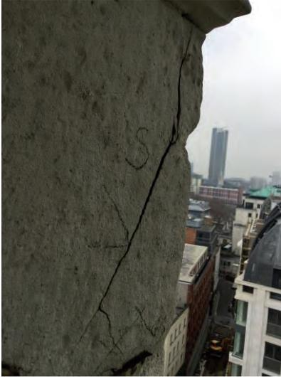
The steeple was inspected again in early February by a specialist team of steeplejacks, they climb the exterior of the steeple, looking for signs of further damage and degradation of the 1719 structure. We are now awaiting their report of the current condition and hope the cold winter has not caused further serious damage.
