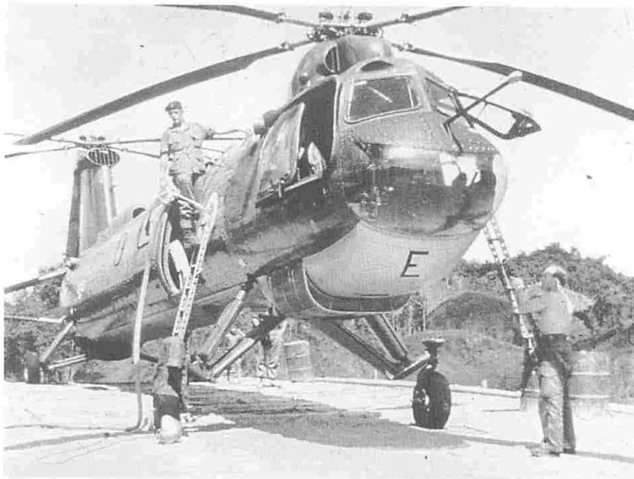
Re-fuelling the front tank of a Belvedere at a forward base in Borneo. Note the proximity of the front engine jet pipes to the re-fuelling airman, and the fuel dipstick which passes through the rotor disc.
