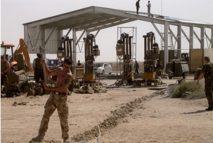
Aircraft shelters being erected on the hardstanding.
