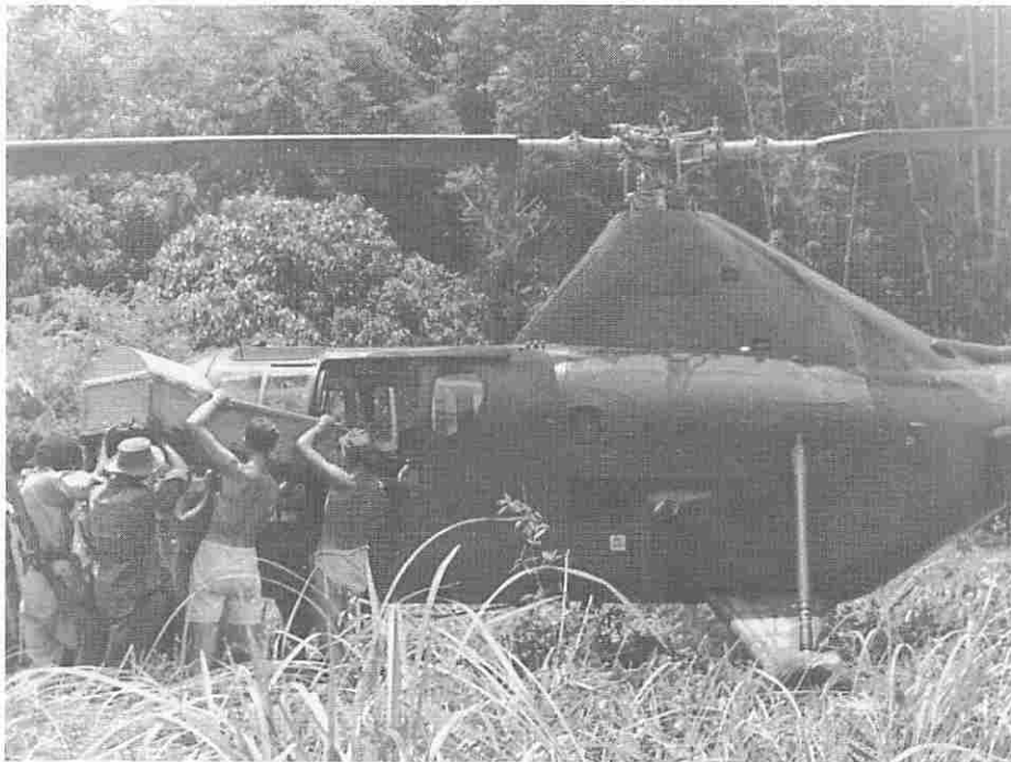
The Dragonfly basket stretcher, which replaced the external pannier, being used to load a casualty in North Malaya in 1952.
