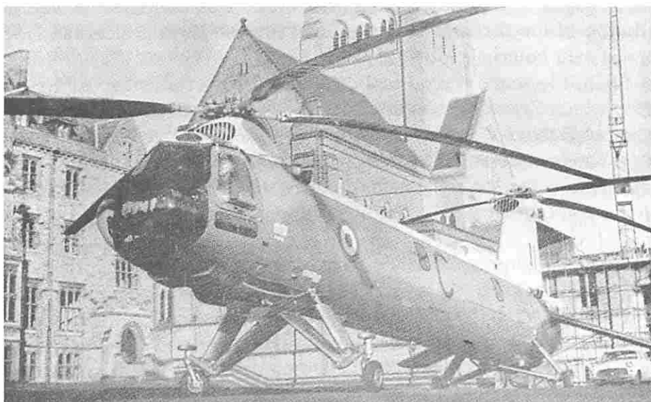
The Bristol 192 pre-production version of the Belvedere with two Napier Gazelle turbine engines and four bladed rotors, but still with wooden Sycamore blades and fully manual controls: used for service trials. (In the background: Ampleforth Abbey.)
