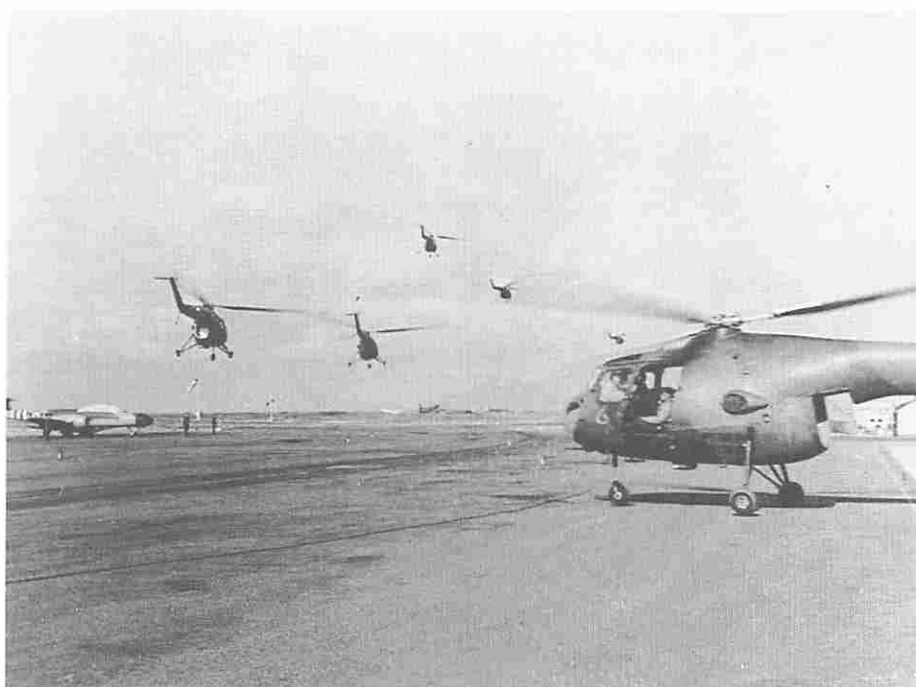
Sycamore troop lift from Nicosia—Cyprus. Baggage and cabin doors have been removed. Note extra passenger carried by rotating the co-pilot's seat to face aft.
