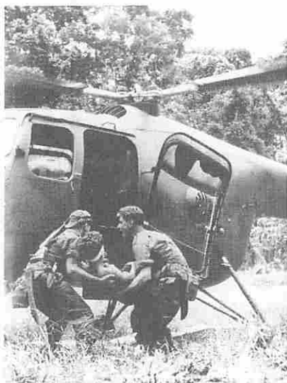
The Mk 14 sycamore could carry 2 stretchers athwartships (but rarely used the upper stowage). A stretcher was sometimes not available and had to be manufactured 'on the spot'. The passenger doors enlarged in the Mk 14 to facilitate stretcher carriage are clearly shown.
