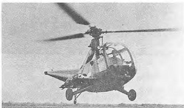
The Sikorsky R-6, which entered RAF service in 1945 as the Hoverfly II: here being flown by Major N Gow of No 1906 AOP Flight. Note the central collective lever; the pilot must sit on the opposite side from the stretcher which has to be on the starboard side because of cyclic control limitations.
