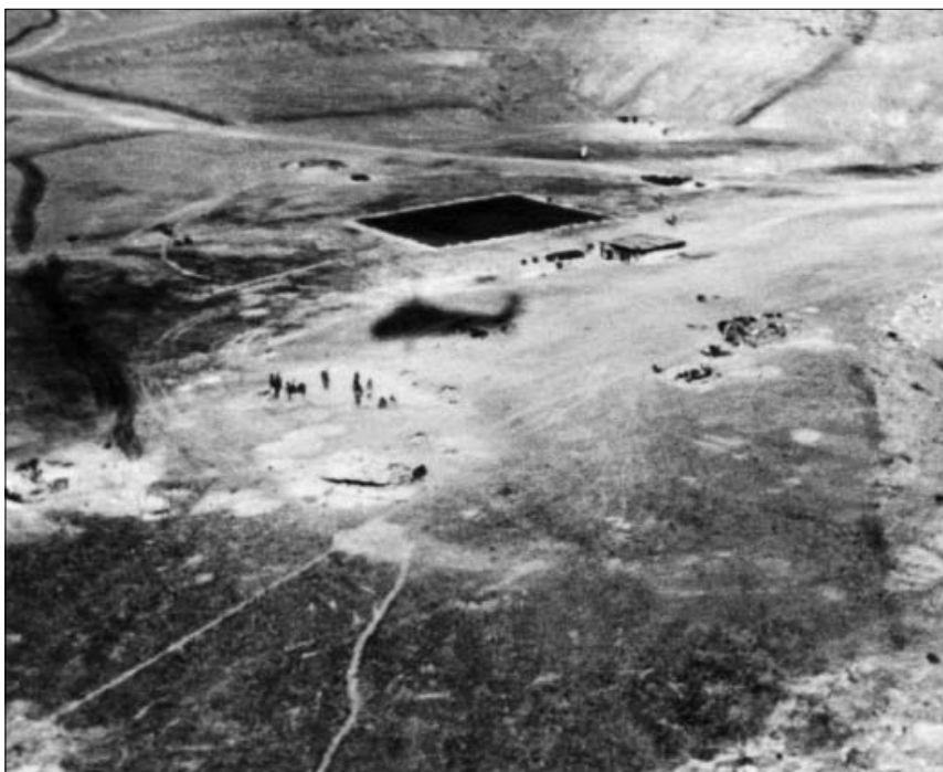
The shadow of a Wessex close to a Dhofar landing zone that has been covered by a neoprene membrane to protect the aircraft from dust and sand
