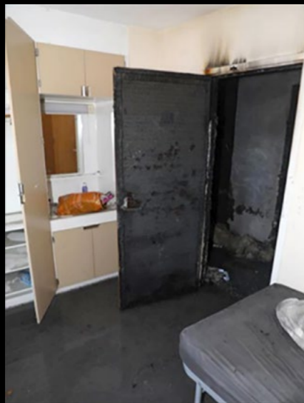
Examples of how fire doors worked brilliantly in the Boulmer SLA fire
