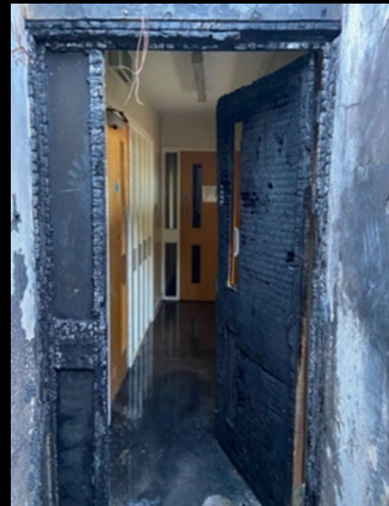
Examples of how fire doors worked brilliantly in the Boulmer SLA fire
