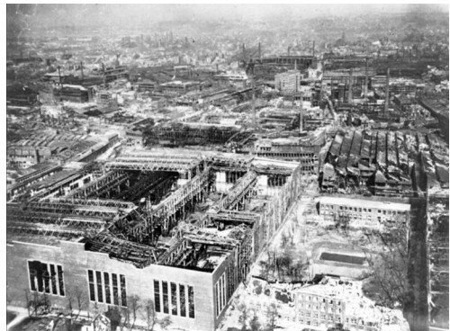
Bomb damage in the Ruhr
