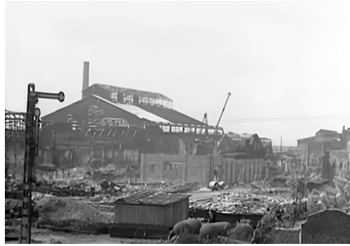
Bomb damage at Bochum Steelworks
