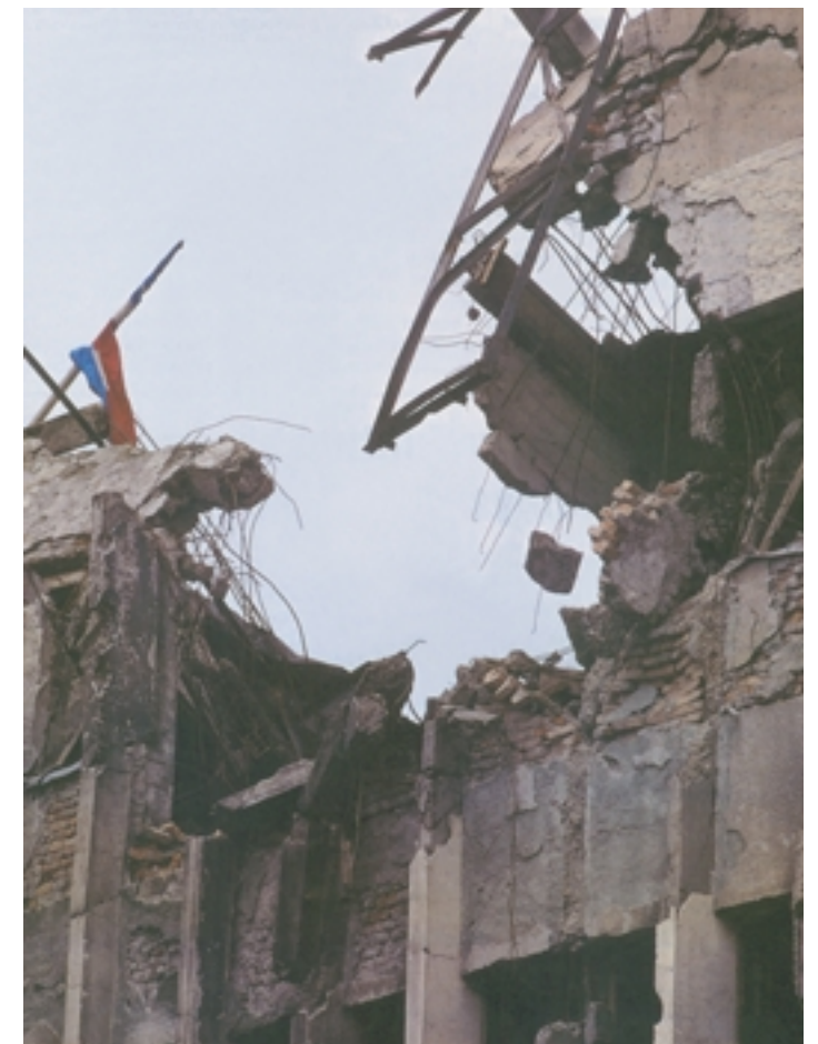
The telephone exchange at Pristina destroyed by a Laser guided bomb.
