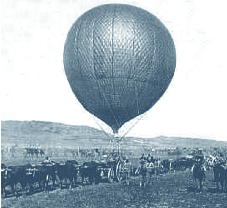
Military balloons varied in size but the 10,000cu ft balloon was typical. They operated at heights of 1,000-1,500ft, in winds up to 25mph. Their role was primarily observation
