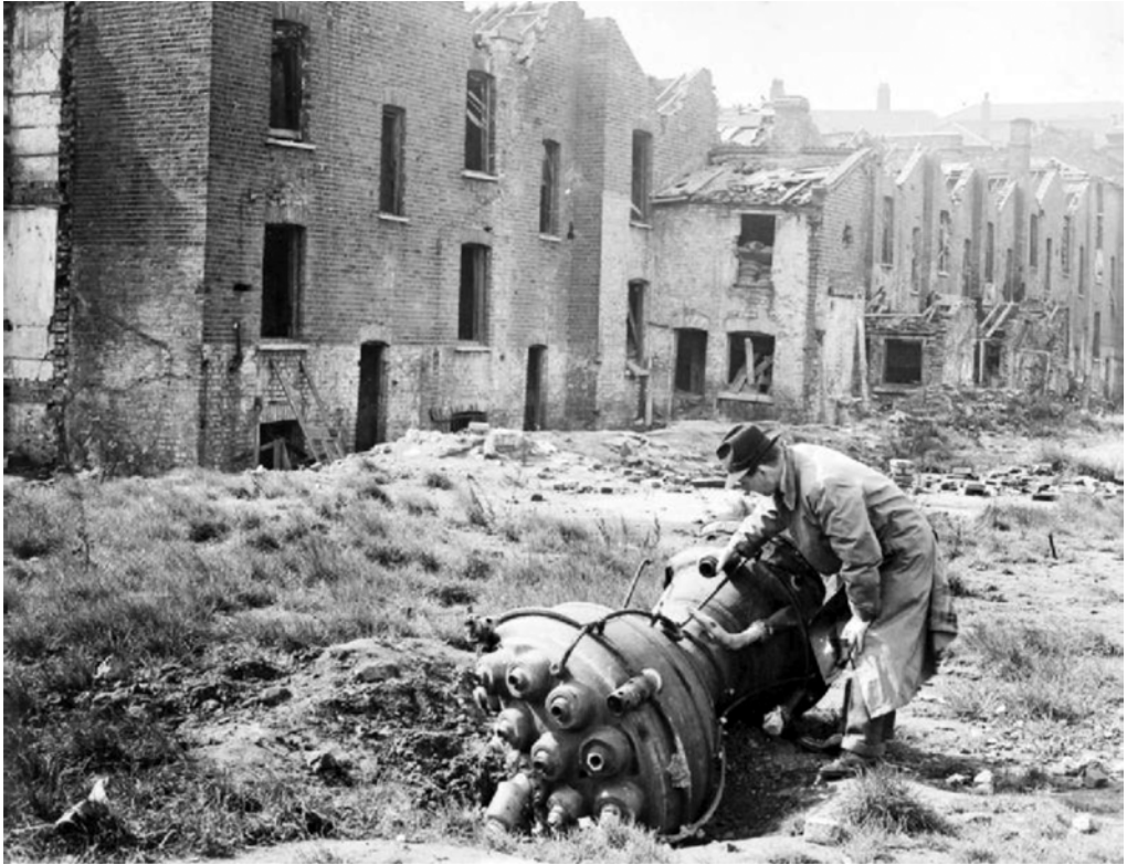
Chinatown (Limehouse, East London) V-2 combustion chamber and venturi which separated from missile on impact. March 1945. http://www.wikiwand.com/en/Limehouse_Causeway
