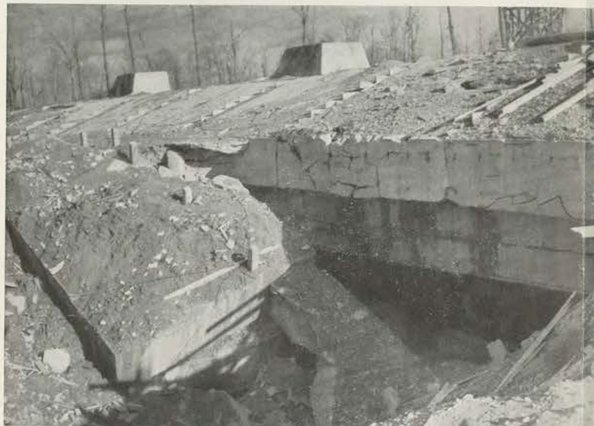
FIG. 31.—SIRACOURT. Vertical photograph of the supposedly "bomb-proof" concrete structure after a direct hit by a 12,000-lb. bomb (arrows).
