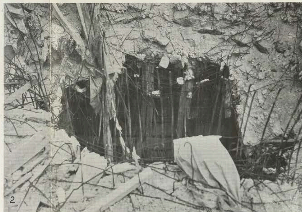
FIG. 37.—BREAST submarine pens. This photograph, taken on the roof of the pens, shows a hole in the 16-ft. reinforced concrete roof resulting from a direct hit by a 12,000-lb. bomb.
