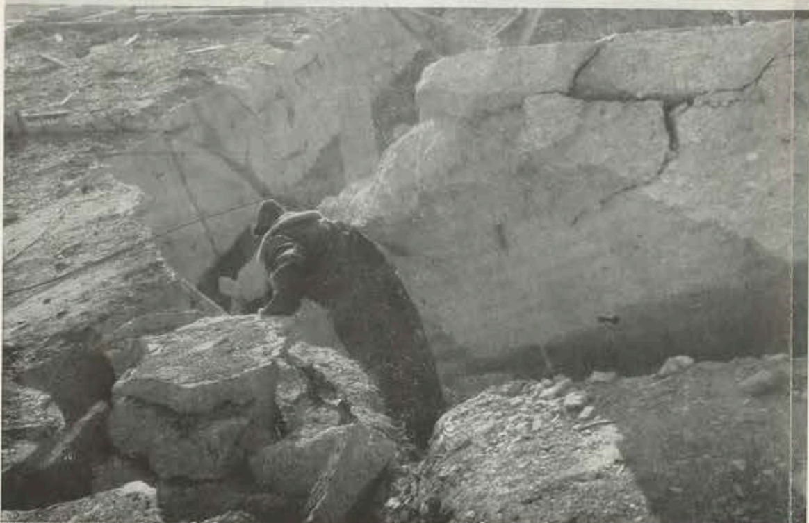
FIG. 32.—SIRACOURT. Ground photographs of the effect on the concrete structure of a direct hit by a 12,000-lb. bomb (compare Fig. 28 above).
