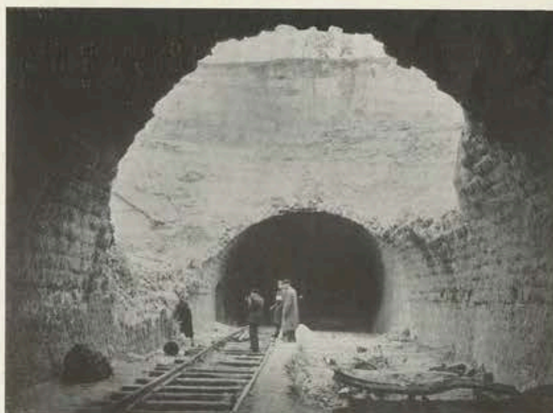
FIG. 2.—SAUMUR Tunnel from within. The damage caused by a 12,000-lb. bomb, as seen after the Allies had cleared the fallen earth and masonry. A vertical photograph of this incident appeared as Fig. 12 in B.C.Q.R. , No. 9.
