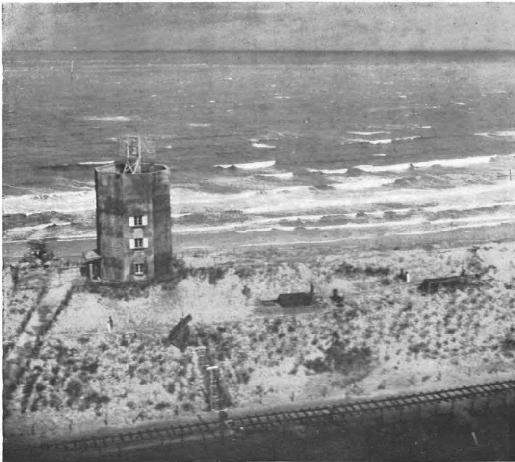
Coast Watching Radar Station at Hook of Holland, showing details of frame aerial array from which it is possible to discover the type of emissions which this station sends out. It would not be possible to find this out from vertical photographs. See letterpress, pages 20-21.
