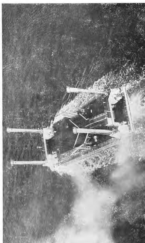
During the invasion the problem of providing port facilities before a major harbour had been captured was partially solved by towing pre-fabricated parts across the Channel and creating an artificial port off the beaches. The photographs on this page were taken by a Swordfish of 819 Squadron (F.A.A.) in June. The upper pictures show concrete caissons for forming breakwaters, and the lower ones show pier-heads for use at the end of floating roadways.
