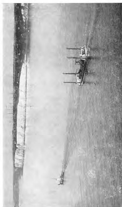
During the invasion the problem of providing port facilities before a major harbour had been captured was partially solved by towing pre-fabricated parts across the Channel and creating an artificial port off the beaches. The photographs on this page were taken by a Swordfish of 819 Squadron (F.A.A.) in June. The upper pictures show concrete caissons for forming breakwaters, and the lower ones show pier-heads for use at the end of floating roadways.
