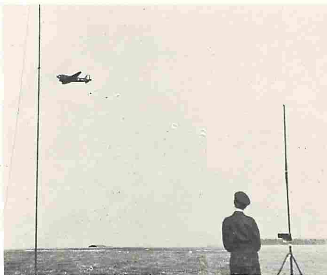
A Dakota dropping ordnance stores on 18 ft. cotton parachutes. In the foreground (right) is the velometer, an instrument for measuring windspeed on the dropping zone for paratrooping operations
