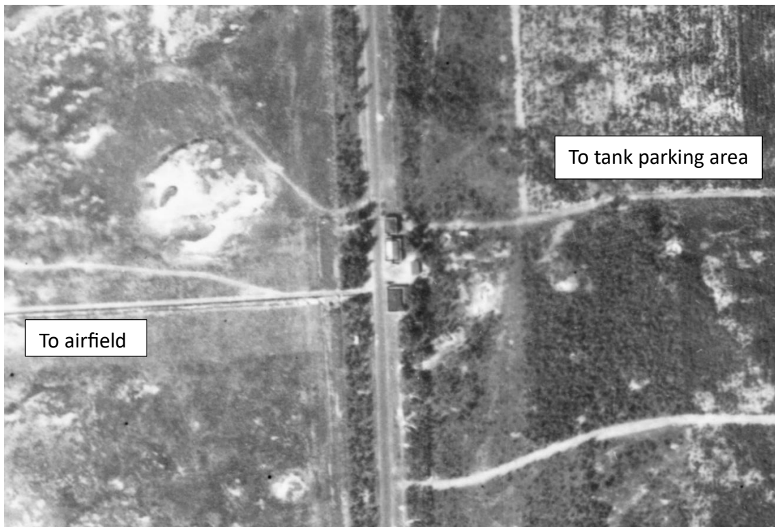
The buildings on the boundary of the Deelerwoud and the airfield.
